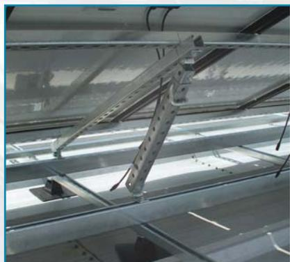
Hex-head bolt threads easily into a spring nut, connecting fitting to channel in a quick one-hand operation.
