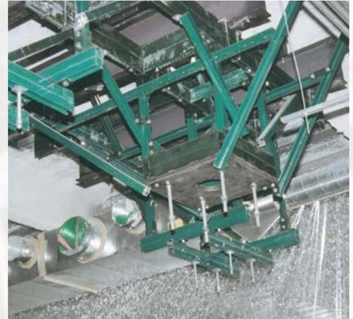
*Final adjustment can be made after all components are in place, to assure precise horizontal alignment.*
